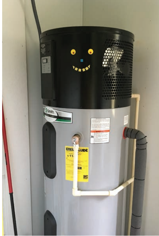
Left: Bruce in the Scionwood Retreat's country kitchen. Right: Meet Omar, our heat pump water heater. Kathryn stuck some magnetic pieces from a magnetic game and created the face on the water heater before she named it. We set the unit to operate only in heat pump mode. Omar saved enough kWh to make room for our charging the Bolt EV without a noticeable jump in our kWh consumption.
