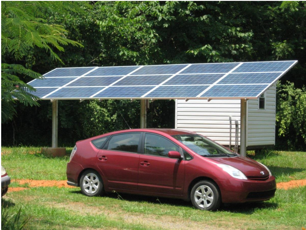
3.5KW pole mount with battery backup 2011
