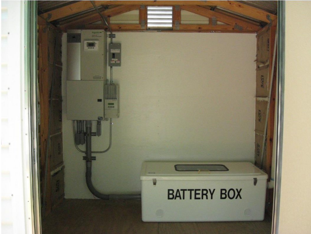
Solar power management system and battery storage
