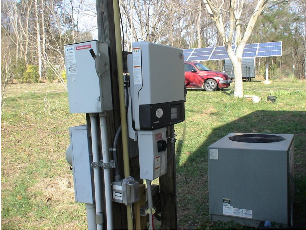
Roof mount solar controller with pole mount in background
