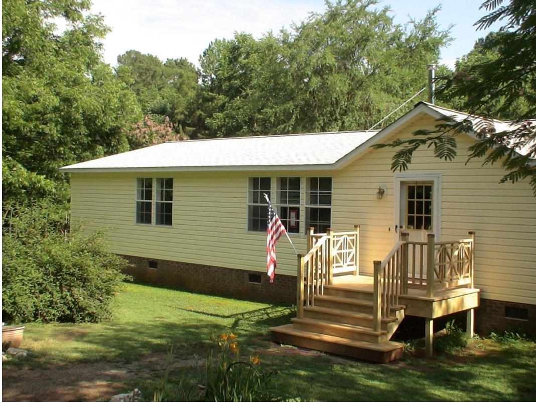
Front of Scionwood Retreat
