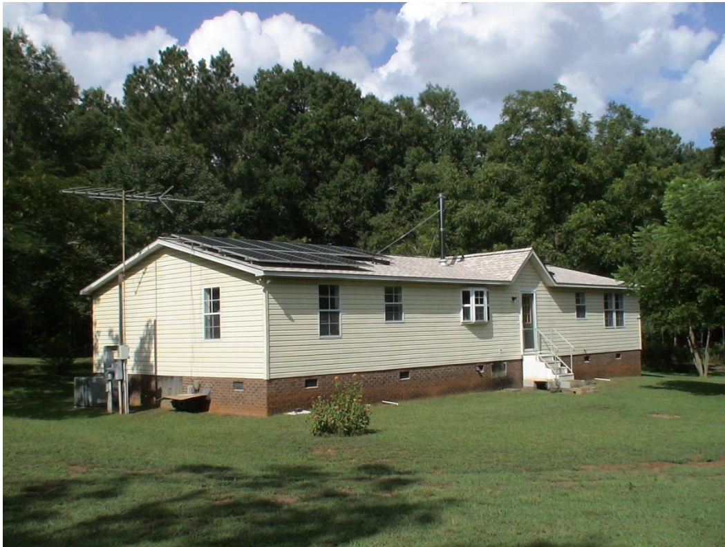
3.4KW roof mount 2015
